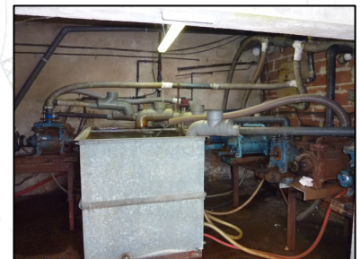
Picture 3 - Previous liquid ring system
