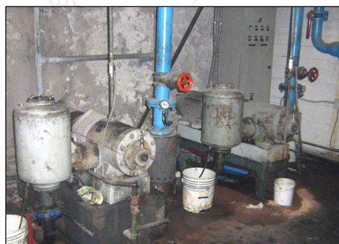
Two Water Cooled V45 Pumps from 1963
