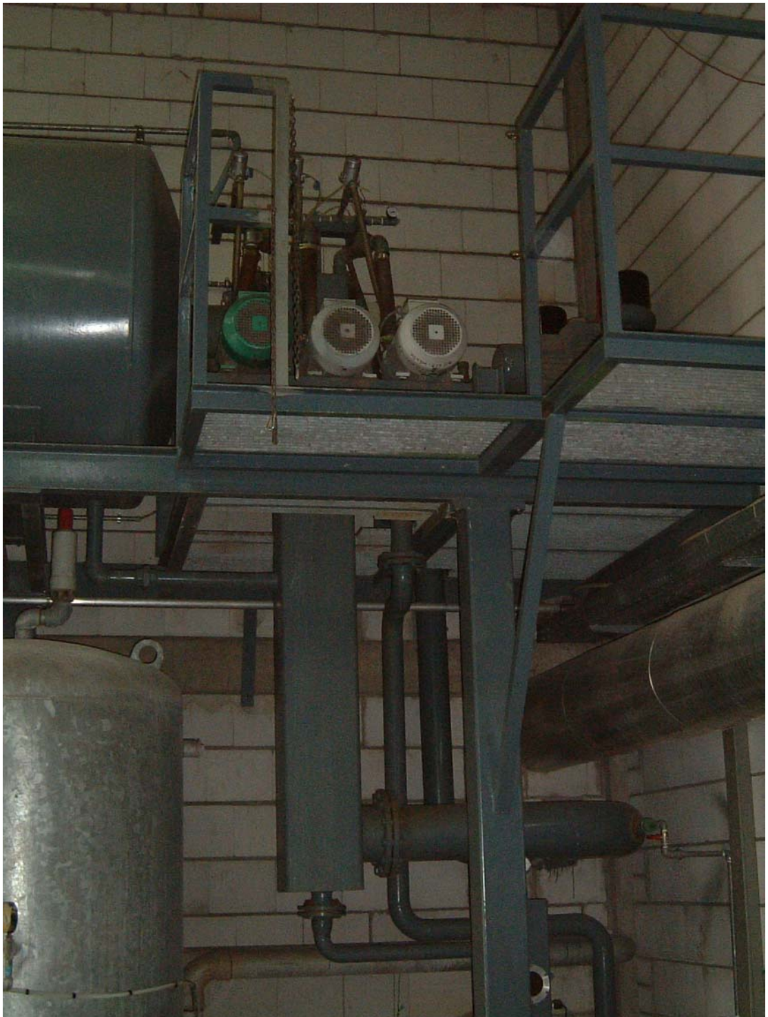
Installation Wasserringpumpen
