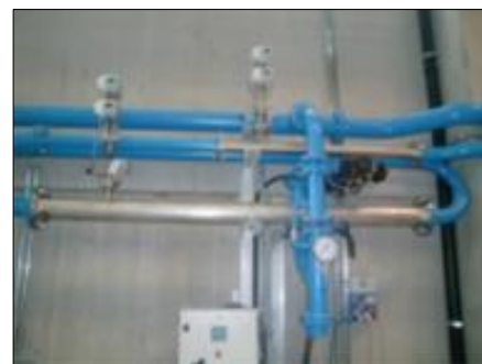
2 measuring tubes (stainless steel) DN 80 and DN 150 with two PoetterSensors® and two DP- Transducers for each pipe
