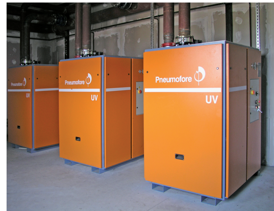
Pic. 3 - Installation of rotary vane vacuum pumps mod. UV16
