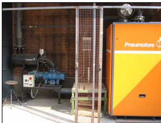
Sicme Motori processes the windings of electrical motors in a receiver of 23 m<sup>3</sup> volume. To guarantee the leak-free operation of the receiver, a gasket filled with compressed air is used. The customer sets the target of minor evacuation time in order to achieve higher productivity.
