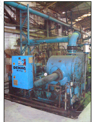
Replaced Wittig WPSO Pumps
