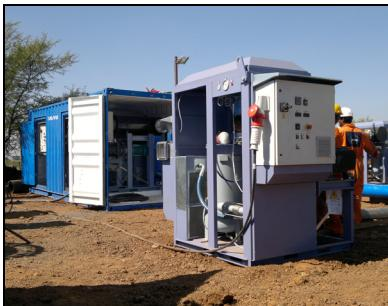
The vacuum drying method was applied after the dewatering with pigs. The considerable volume of 102.000 m<sup>3</sup> was evacuated down to 0,3 mbar(a) [29,905 in Hg (V)], which corresponds to the Dew Point of -32° C [-25.6° F] in 6 days only.
