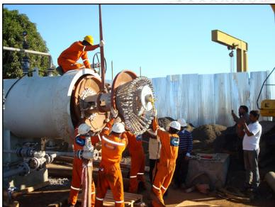
During the commissioning, the Pneumofore engineers instructed the local team about the vacuum pumps operation and maintenance. The routine operations on the vacuum systems, as well as the periodic checks, are fast and simple. The air cooling was particularly appreciated due to the critical availability of cold water for cooling purpose.
