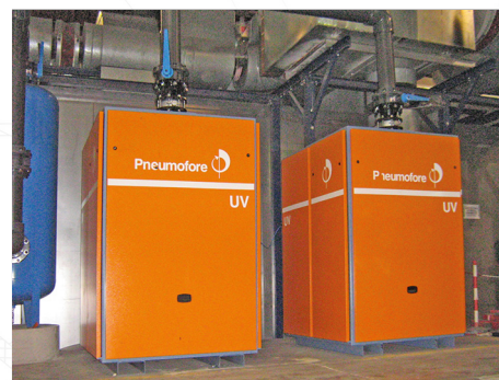
UV16 vacuum pumps installed at Crown in 2006
