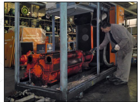
UV30 dismantling and cleaning
