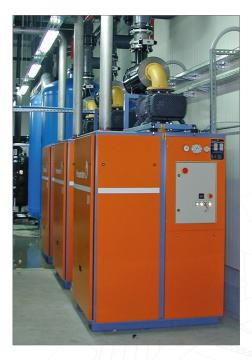
To meet the increasing demand for the packaging of sliced meat and other perishable foods, centralized vacuum solutions replace systems made of multiple small vacuum pumps and reduce oil exhaust and noise levels in the production facilities.
