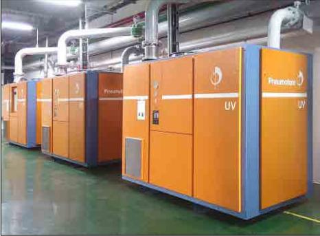
Vacuum is used in the majority of container glass plants, especially on the blow side of the IS machines. This is now also the case of the Rojana plant of Siam Glass, which is testament of Pneumofore's commitment to vacuum implementation for higher machine speed and lighter bottles. Practically, each day 21.600 more bottles and weight reduced from 145 to 140 gr.
