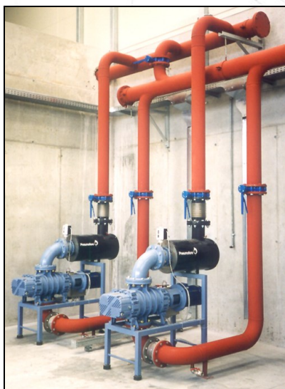
Second stage Pneumofore roots pump
