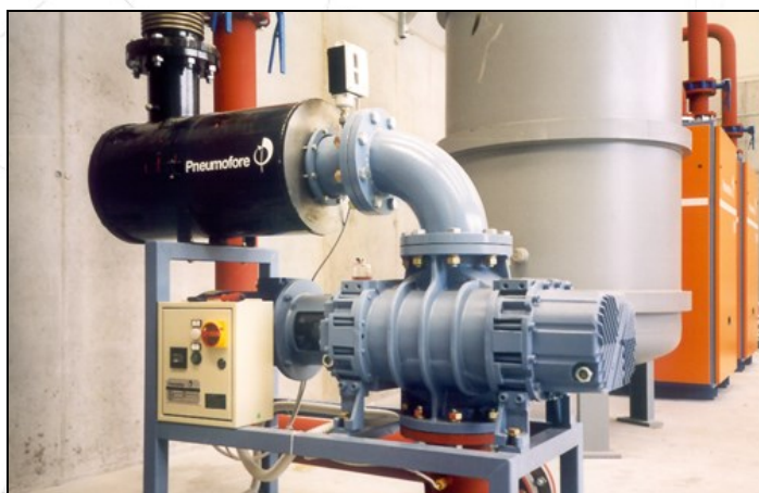
Second stage Pneumofore roots pump, detail of custom installation
