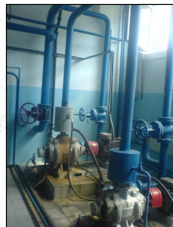
Fig. 2 - Liquid ring pumps
