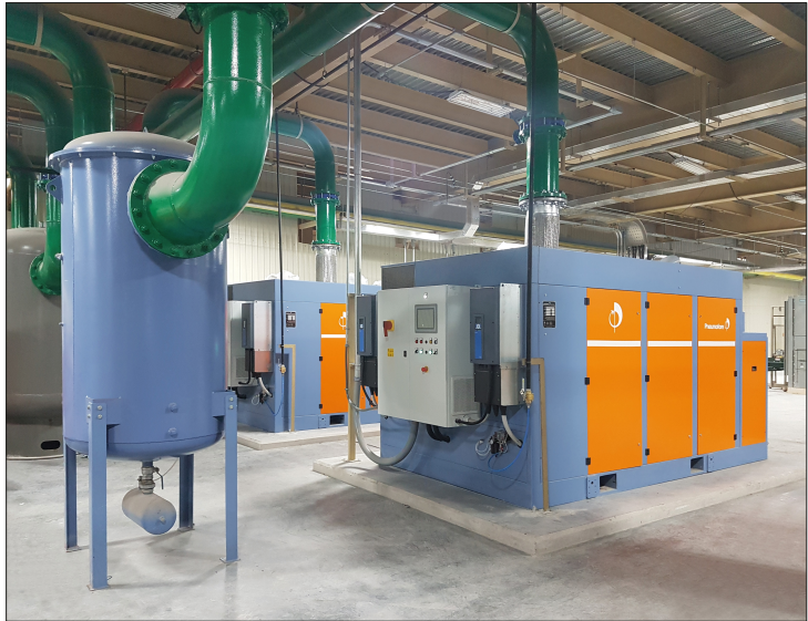
Pneumofore UV100 Vacuum Pumps in Industria Vidriera de Coahuila (IVC)
