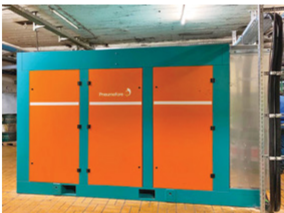
The Pneumofore A400 Air Compressor installed at Weck Glaswerk.
