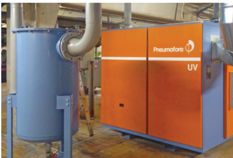
Pneumofore UV30 Vacuum Pump with Variable Speed drive.
